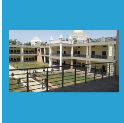
Stainless Steel Handrails
